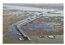
construction of a storm surge barrier and permanent closure of the Outlet to maritime shipping in April 2009. The photo shows the surge barrier under construction. The GIWW is in the foreground, the MRGO in the background.
